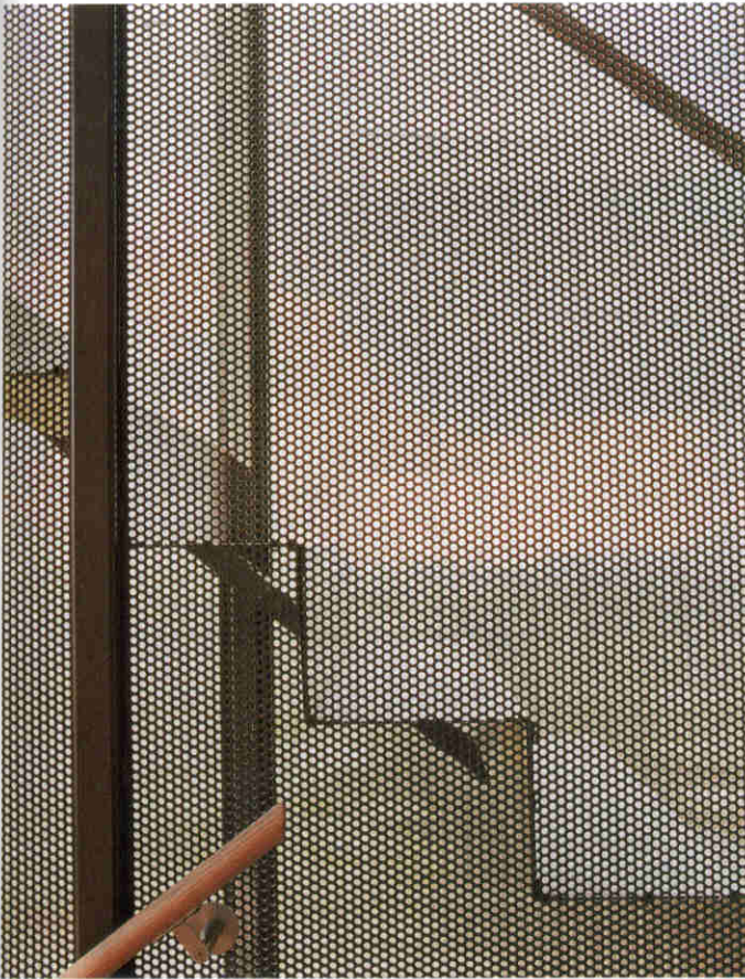
Metal casing Perforated metal forms a semi-transparent casing for the stairs. Inside, the stair treads are as simple as possible so that the overall appearance through the metal is clean and unfussy. Try cadisch.com for perforated plates.
