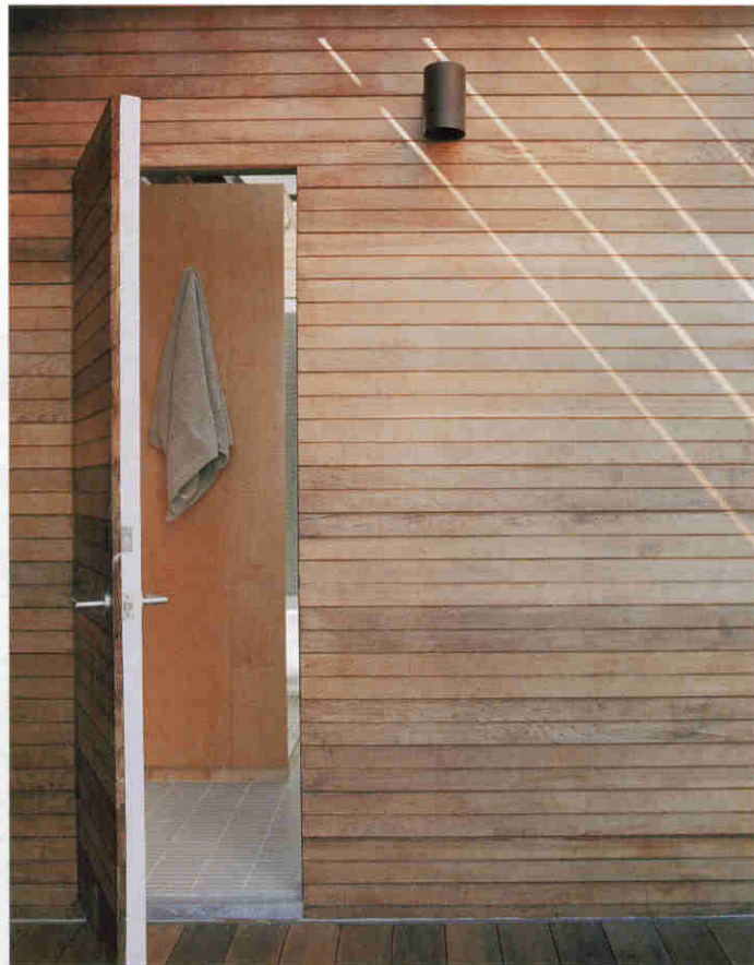
Wood panelling Cedar clads the walls, while the floor decking is made of tigerwood. All of the wood in the house is FSC-certified. Finnforest ( finnforest.co.uk ) supplies various sustainably managed timbers.
